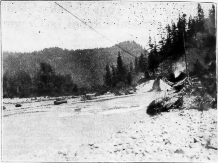
Showing the Path of the Five-Yard Bucket
